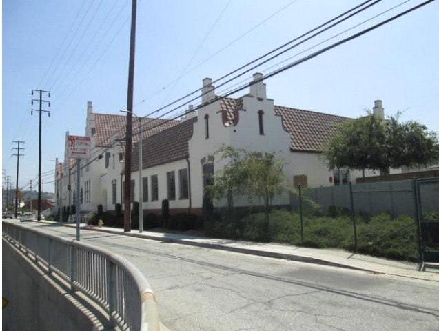
View of bakery building looking northeast, 7/7/16
