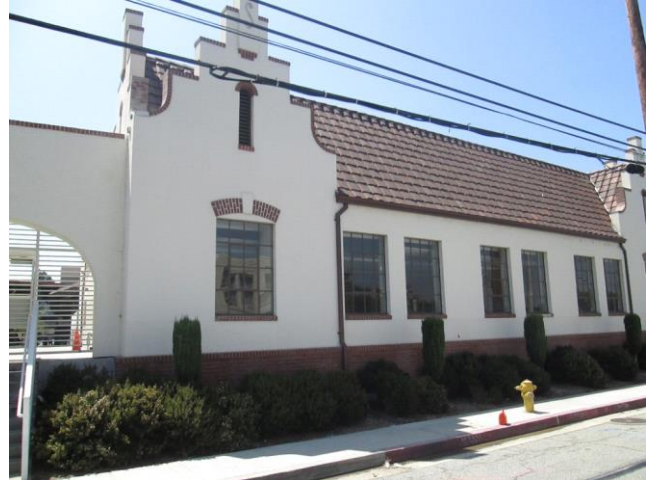
View of receiving building looking southeast, 7/7/16
