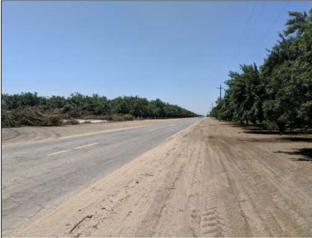
Photo 1. Typical view of sewer pipeline alignment conditions. Photo taken along Riverside Avenue.
