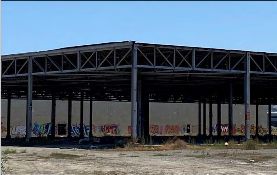
**Photograph 6. Detail of steel framing used in 1960 constructed manufacturing building remnant (21-0522-01), facing northeast.**
