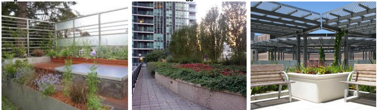
Image 9: Examples of Wind Reduction Measures for Above Grade Terrace Areas
