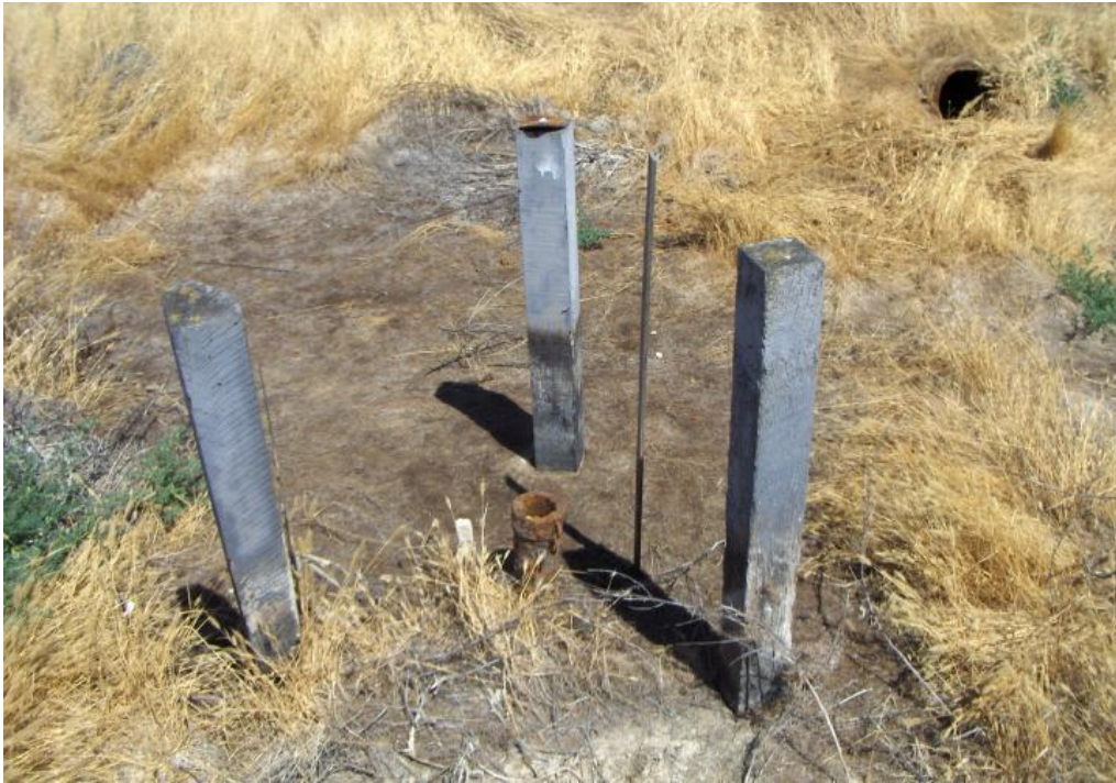
Example of an existing settlement monitor, located at SCPL Site 4.
