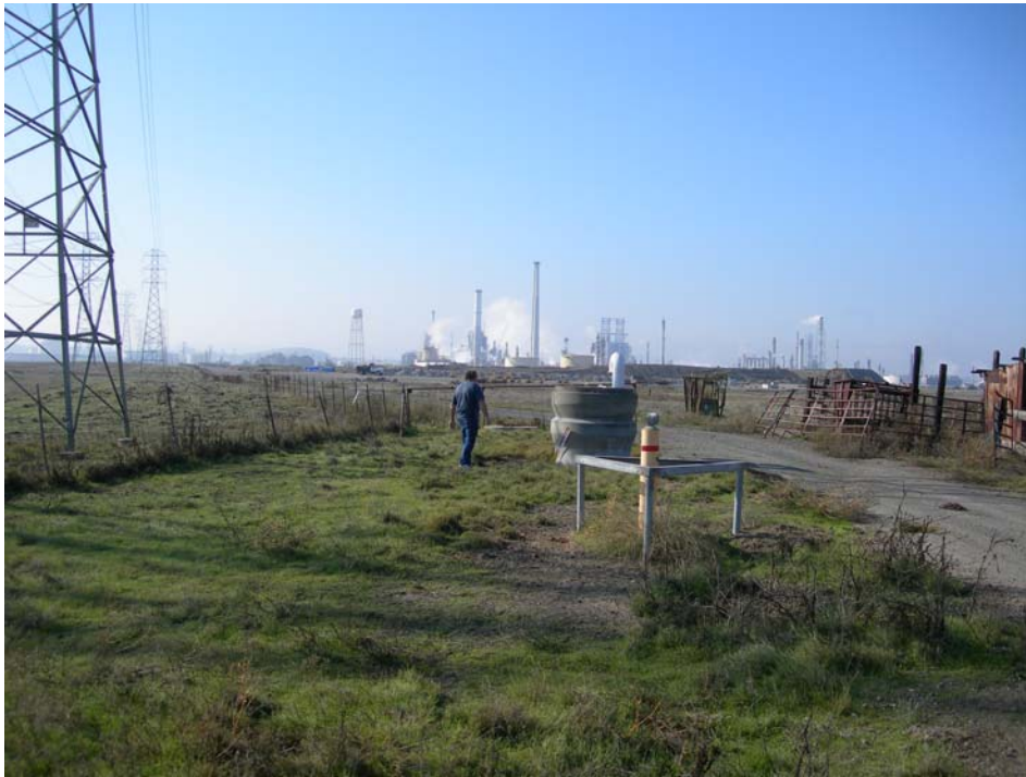
Existing Blow-off Valve located alongside Monsanto Way, looking west toward Tesoro Refinery at Site 9.
