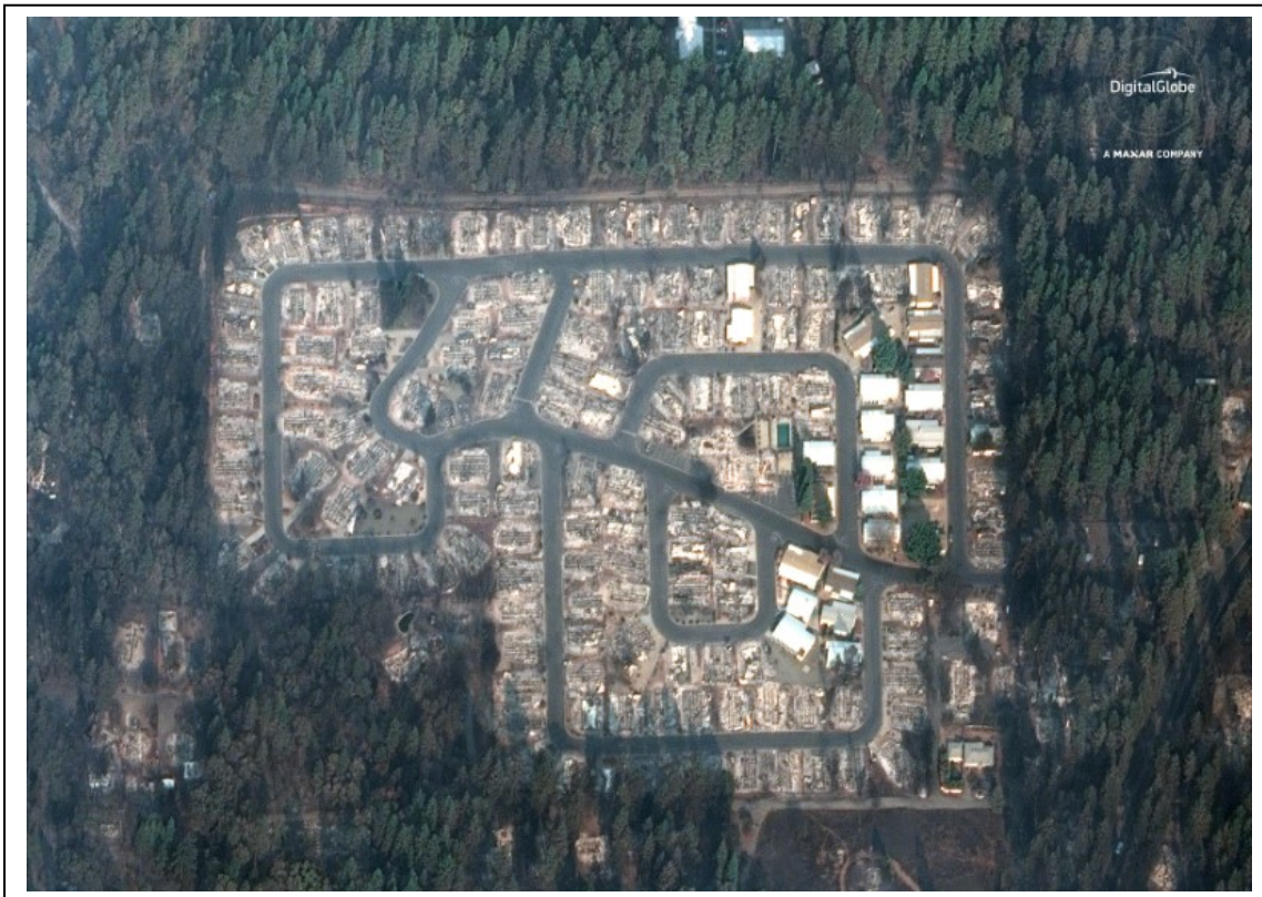
Figure 6 (below). Camp Fire, showing the devastation of homes in the Kilcrease Circle community of Paradise. Note the surrounding green, mature forest with little or no scorching. The homes were not burned by a high-intensity crown fire, but were ignited by embers, followed by home-to-home ignitions. Photo: Digital Globe, a Maxar company via Reuters, 11/17/2018.
