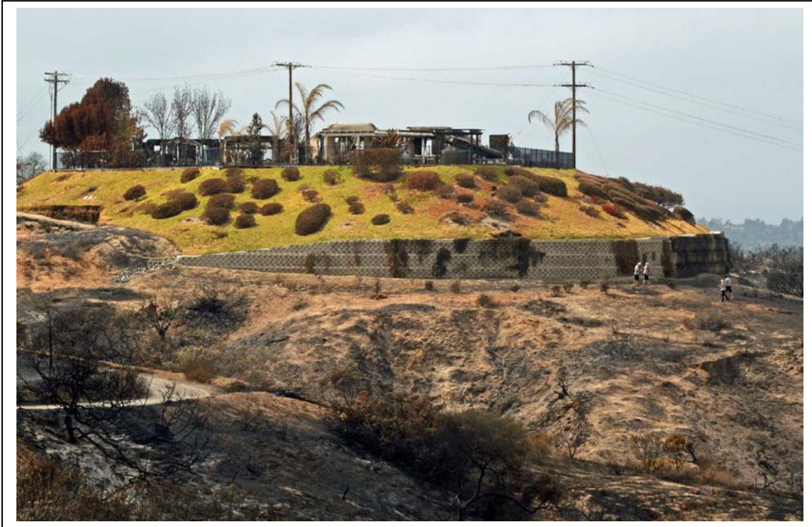
Figure 5 (above). Homes represent one of the most flammable concentration of dead fuels. Despite defensible space, the two homes on this hilltop burned in the 2014 Poinsettia Fire.
