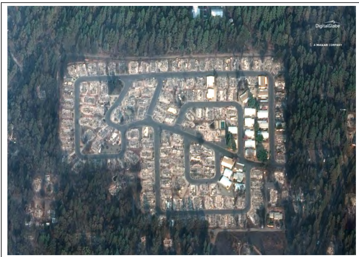
Figure 1. Camp Fire, showing the devastation of homes in the Kilcrease Circle community of Paradise. Note the surrounding green, mature forest with little or no scorching. The homes were not burned by a high-intensity crown fire, but were ignited by embers, followed by home-to-home ignitions. Photo: Digital Globe, a Maxar company via Reuters, 11/17/2018.
