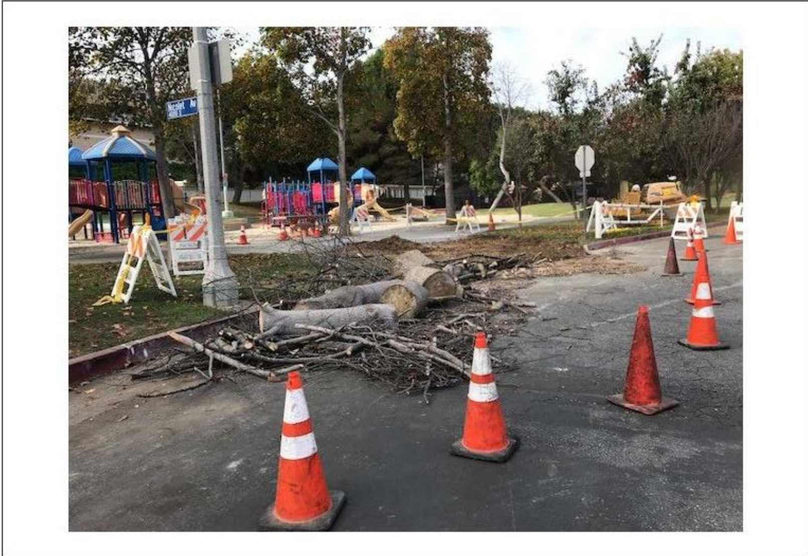
Figure 2-10a. Photo of Construction – Street Tree Removal
