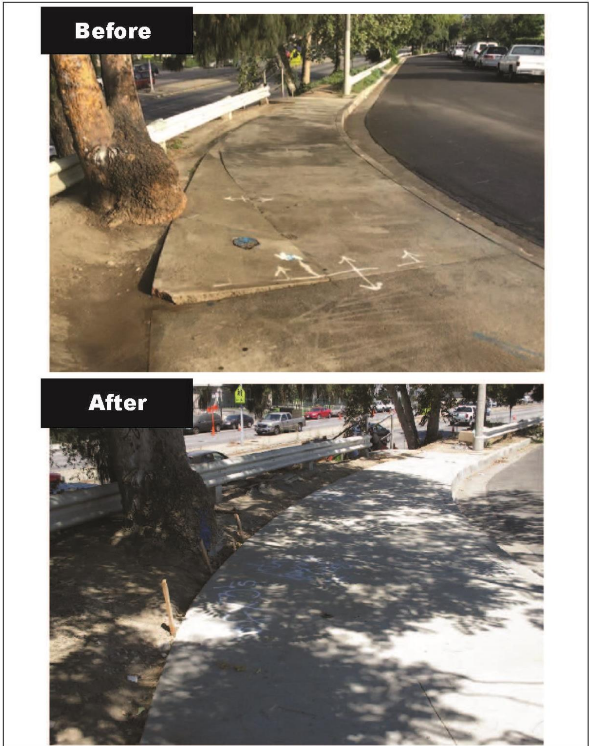
Figure 2-4b. Sidewalk Repair – Before and After
