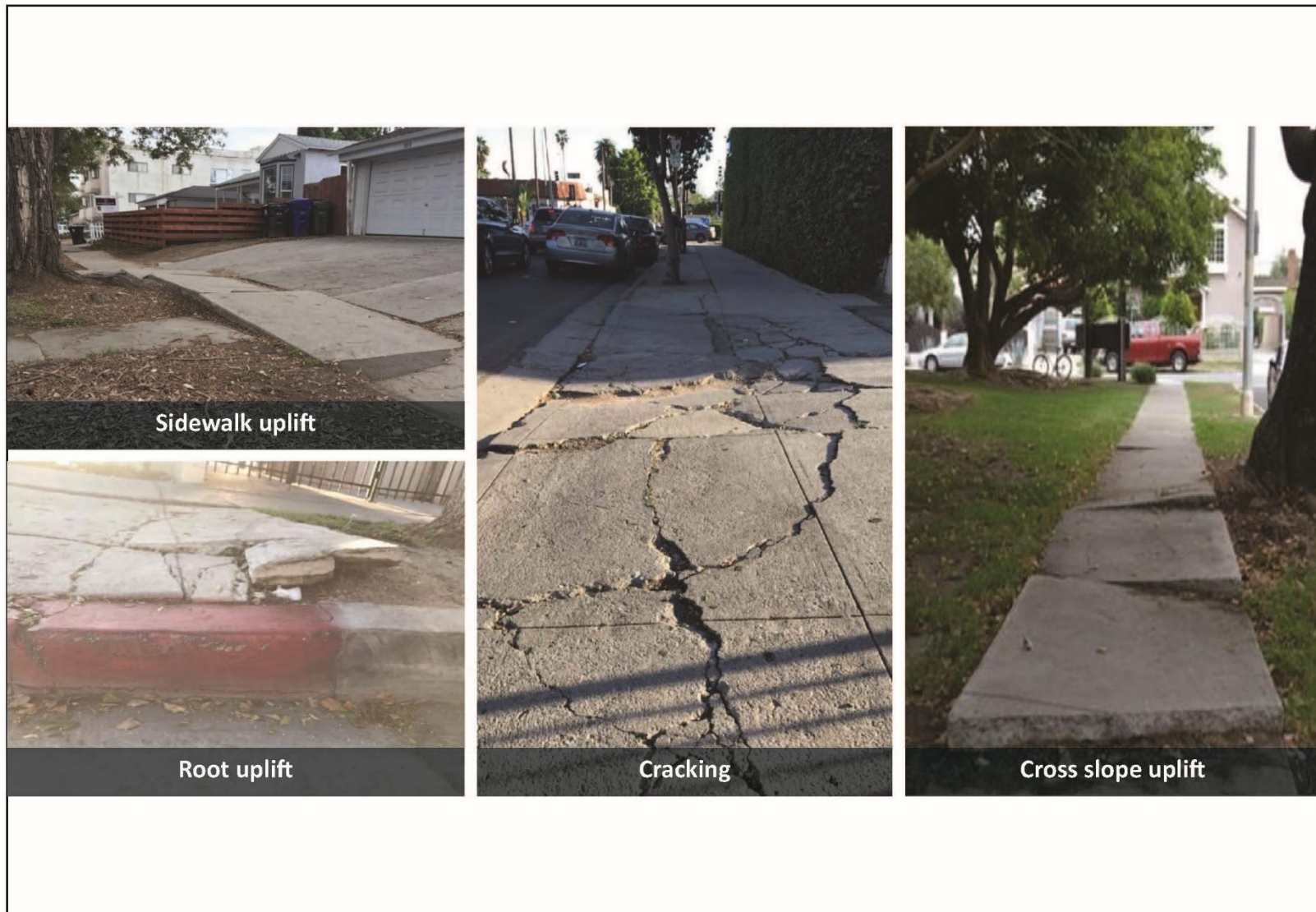
Figure 2-3b. Existing Sidewalk Conditions
