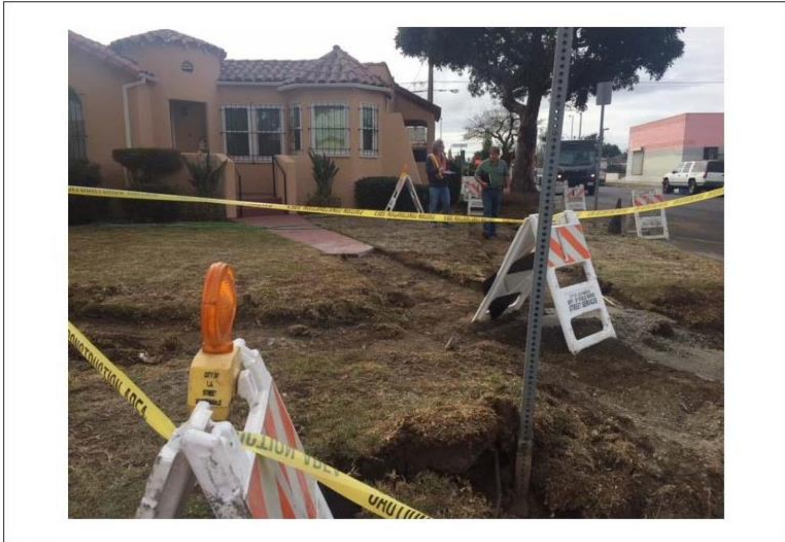
Figure 2-8. Photo of Construction Affecting Private Walkway
