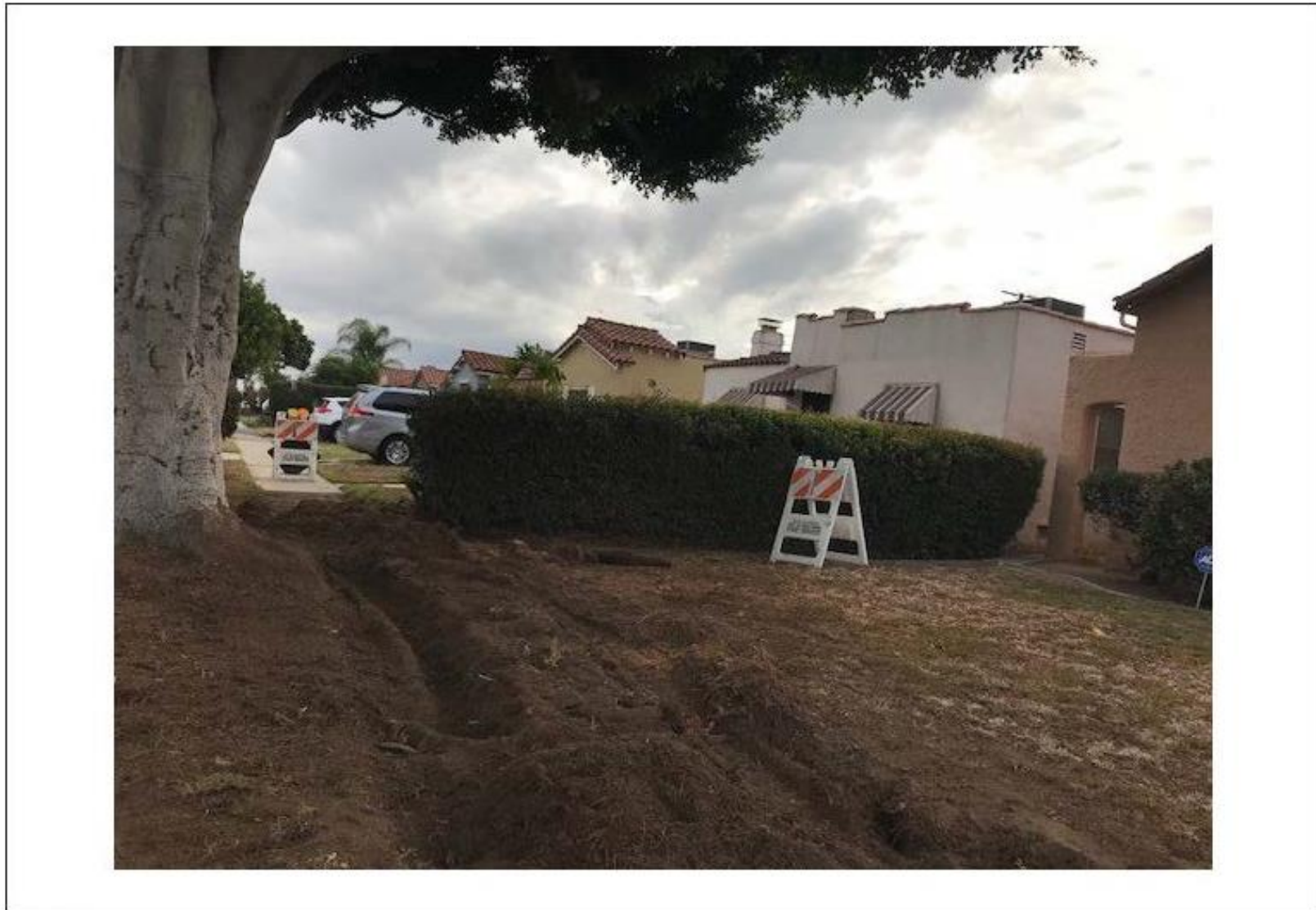
Figure 2-9. Photo of Construction – Street Tree Root Pruning – Existing Sidewalk Removed
