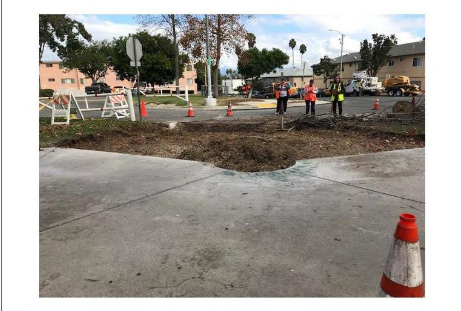
Figure 2-10b. Photo of Construction – Street Tree Removal
