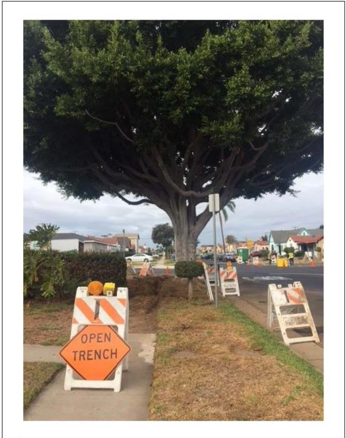
Figure 2-7. Existing Sidewalk Removed and Root Pruning Complete
