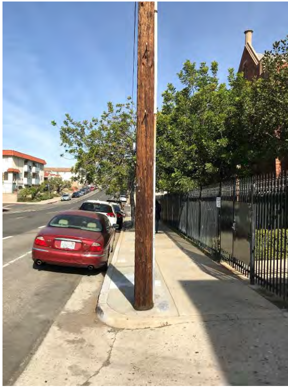
Photograph 37: LT10 Looking North
