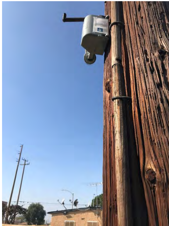
Photograph 36: LT9 Looking West
