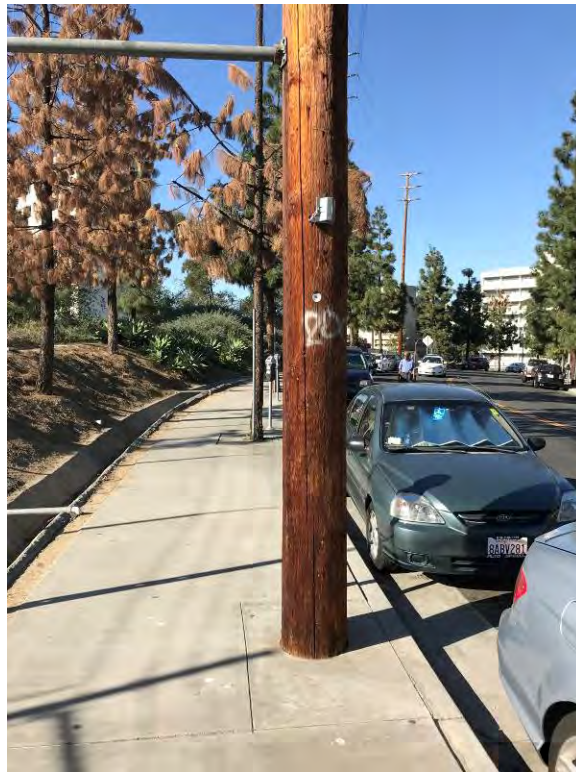
Photograph 28: LT7 Looking Northwest
