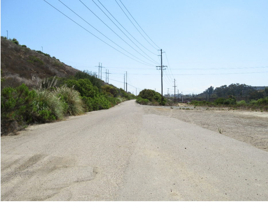
Plate 5. Overview of Carroll Canyon Road extension area, view to the east.
